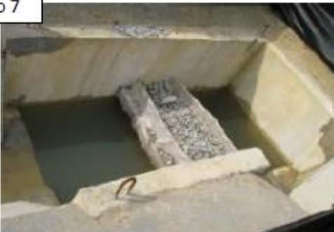
Silt trap are maintained before and after rain
