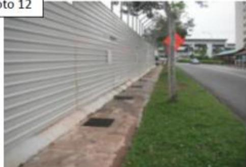
**Bottom of site hoarding sealed with concrete**
