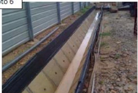
Silt fence and cut-off drain are properly installed
